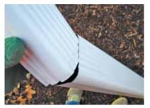
Attach extensions with two short sheet metal screws per joint. To prevent leaks, do not put screws in the bottom of any
