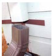
Wrap the downspout strap around the new downspout assembly and attach all three pieces together with two short sheet metal screws.
